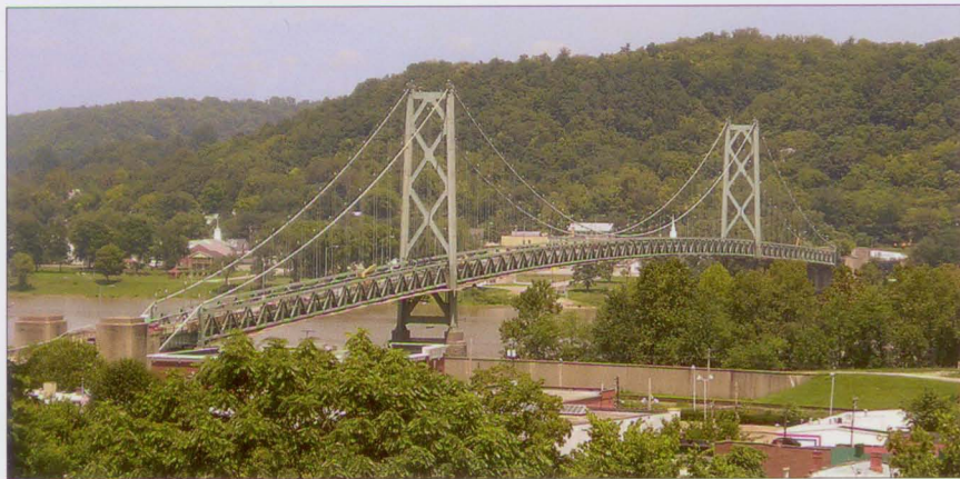
▲ Shortened. Suspension bridge's deck is replaced using fewer stages under alternative plan.
